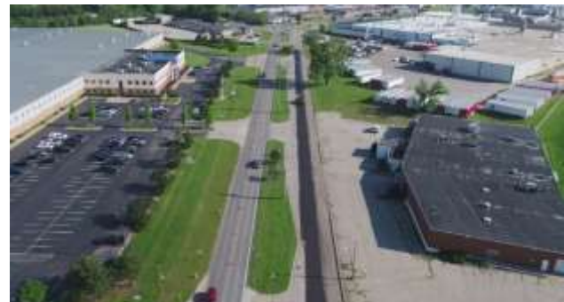
Figure 5. Entrance to the Kerper Boulevard Industrial Park.
