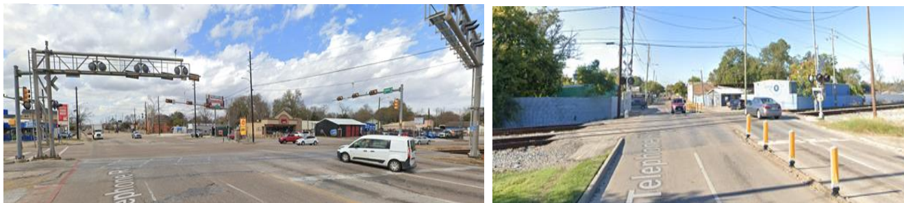
Figure 4-5 Telephone Road at Griggs (Left) and at Tellepsen (Right)
