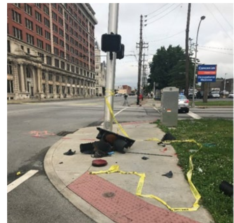
Figure 23: Utilities damaged on 9 th Street
