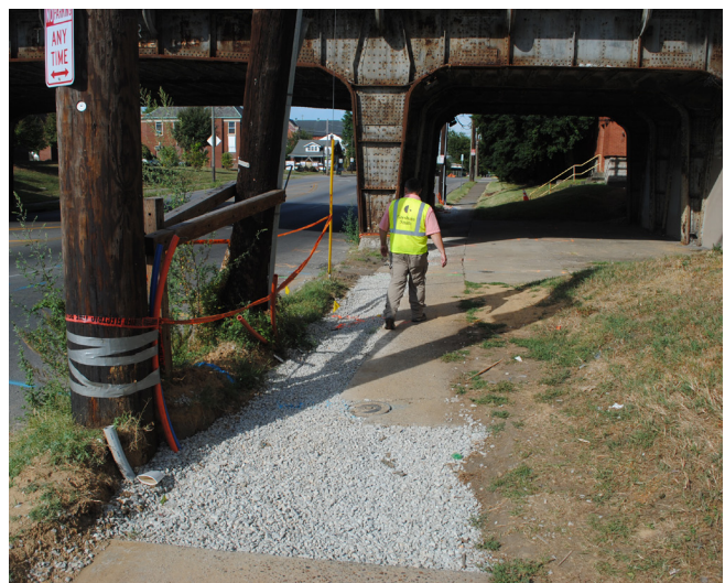
Photos of existing site conditions along the Broadway and Baxter Corridor
