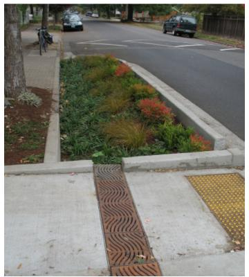
Example of green infrastructure with bioretention stormwater management integrated into the streetscape design
