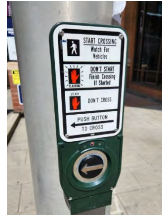
Image 2: An accessible push button for signalized crosswalks, a low-cost improvement.
