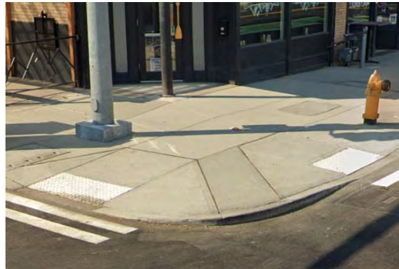
Image 4: Dual curb ramps are the standard for new construction in the City's design guidelines.
